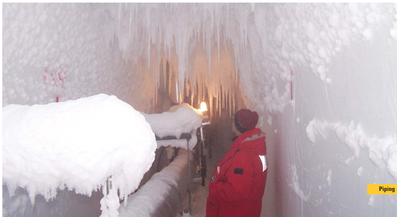
Amundsen-Scott South Pole Station
